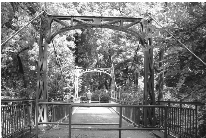
Figure 8. Front view. Iron suspension bridge in the public park of Vilvoorde, 1899.
