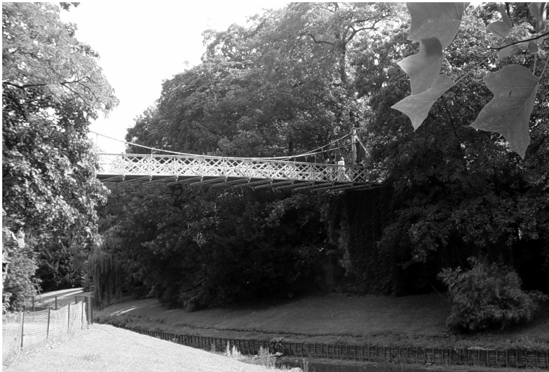
Figure 4. Side view. Iron suspension bridge in the public park in Antwerp, 1869.
