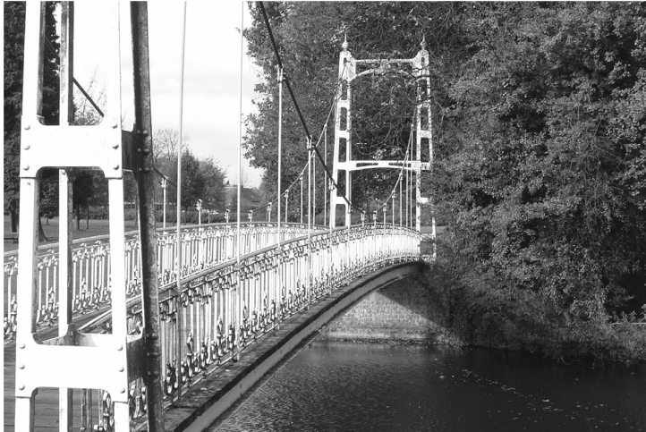
Figure 10. Side view of the iron suspension bridge in Beveren, near castle Cortewalle, 1900-05.
