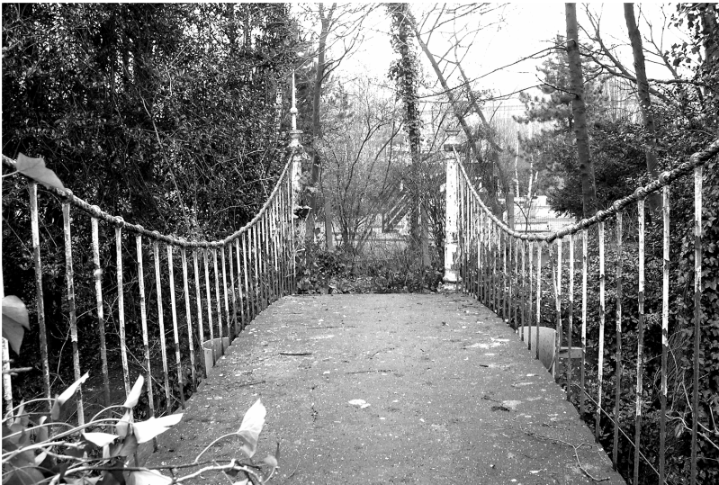
Figure 6. Front view. Iron suspension bridge at the municipal school of Zelzate, 1880-5.
