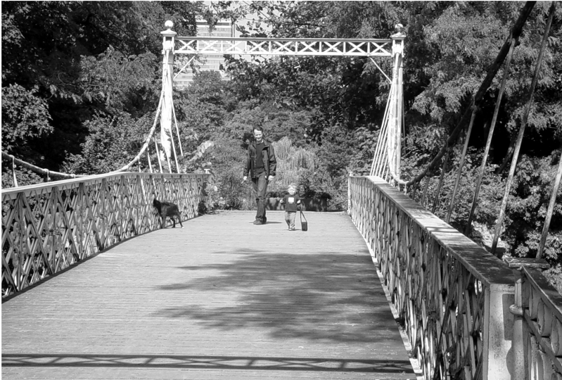
Figure 5. Front view. Iron suspension bridge in the public park in Antwerp, 1869.
