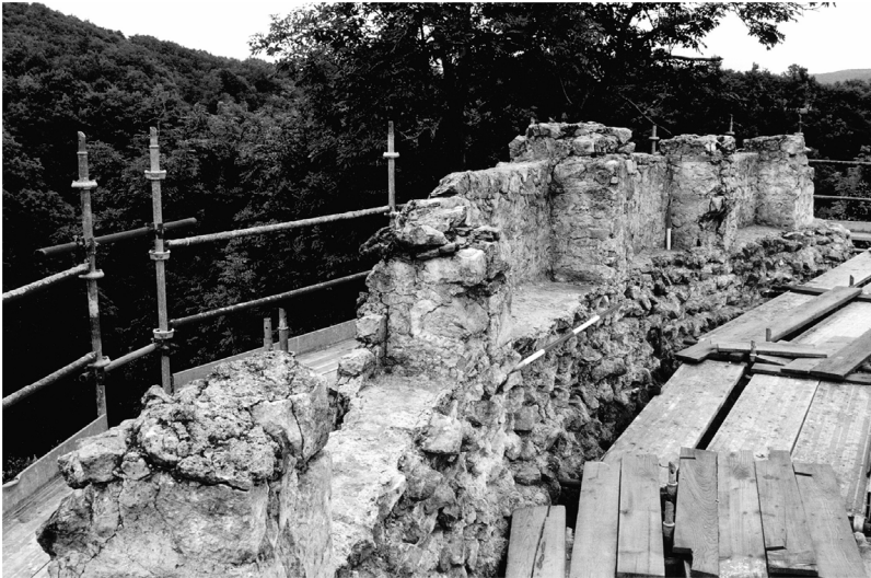
Figure 3. The south-west angle of the defences displays the best preserved Roman fabric. Here both sides of the wall can be seen standing to almost their original heights. Removal of vegetation and later masonry at the top of the wall revealed the exceptionally well-preserved Roman wall-walk, external cornice, parapet and lower halves of five traverses (internal buttresses), as well as evidence for four merlons and three embrasures
