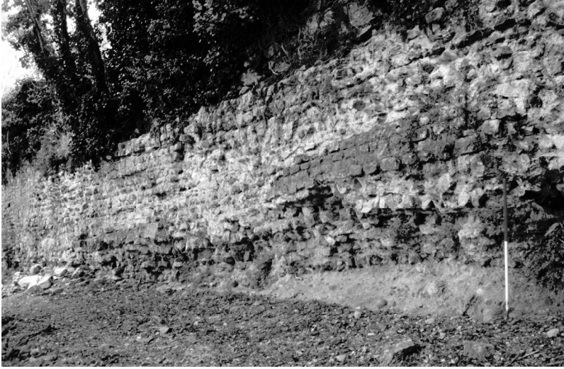
Figure 2. The north-western parts of the defences are well preserved. The Roman fabric is for the most part easily distinguished from that of later periods by its regular, coursed rubble corework or its facing in petit appareil with courses of brick and tile. Note how the foundations are now exposed due to erosion at the base of the wall. Note also how the construction courses follow the natural slope of the ground
