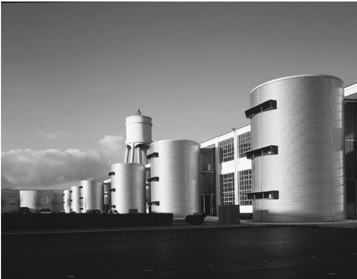
Figure 13. Rear view of completed redevelopment showing new service drums, link corridors and glazing, 2002.
