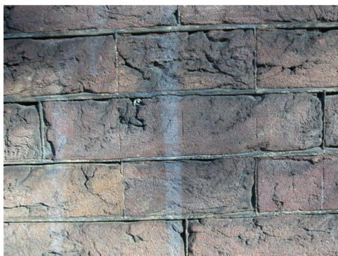
Figure 14. Leiden, façade of 12 Nieuwe Rijn, stretch with marking scratches
