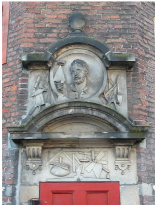
Figure 2. Entrance of the guildhall for the bricklayers, stonemasons, slaters and pumpmakers in the northeast tower, sandstone 1617
