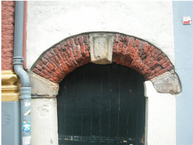
Figure 12. Arch next to 4 Springweg Utrecht, dilapidated gauged brickwork
