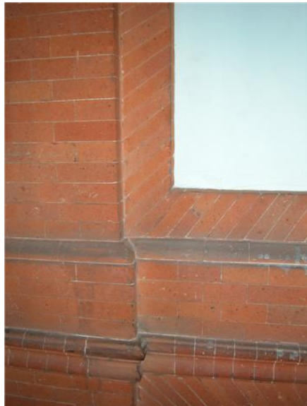
Figure 8. Gauged surfaces of a masterpiece in the guild's meeting room
