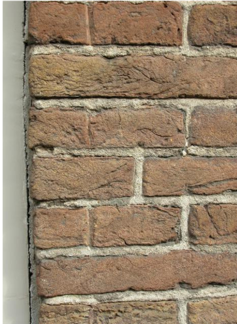
Figure 13. False vertical pointing on three-quarter bricks near an edge in the façade of 15 Koningsstraat Amersfoort (ca. 1685)
