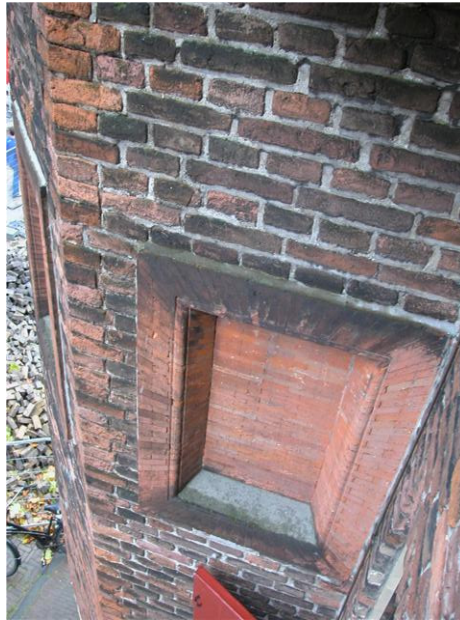
Figure 10. Rubbed corner stones in the northeast tower (1488) with a few gauged masterpieces (17-eighteenth century)
