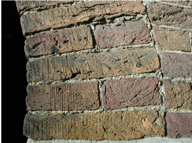
Figure 11. Zijlpoort Leiden (1667-'69) prepared bricks with grooves and hatches at the inside of the gate
