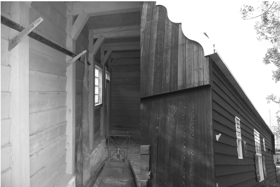
Figure 10. Interior view (left) and exterior view (right) of clapboard siding on buildings in the Zaan region
