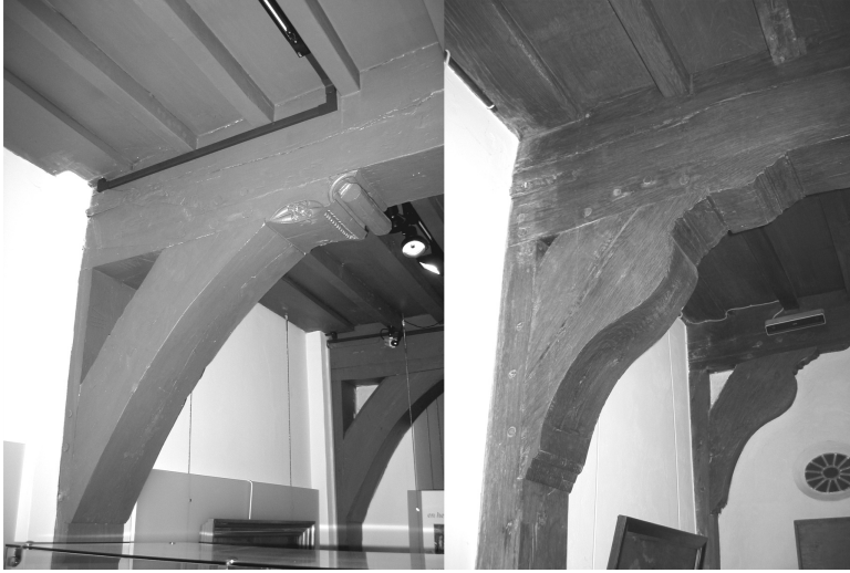
Figure 6. Left a brace with a carved corbel piece ( sleutelstuk ), right an S-curved brace ( zwanenhals korbeel )
