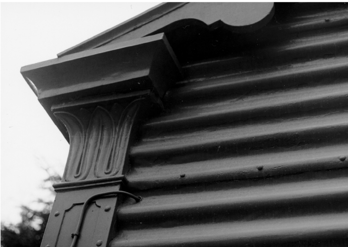
Figure 6. Five inch pitch on horizontal sheeting, Balmoral ballroom
