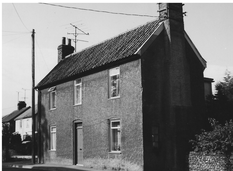
Figure 5. Rectangular two storey gabled toll-house: Claydon
