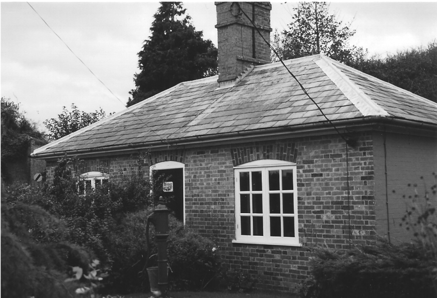
Figure 9. Rectangular one storey hipped toll-house: Wells next the Sea
