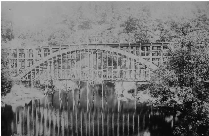
Figure 10. Oliveira de Frades bridge over the Vouga, shuttering, 1906. (IFA/CAA)
