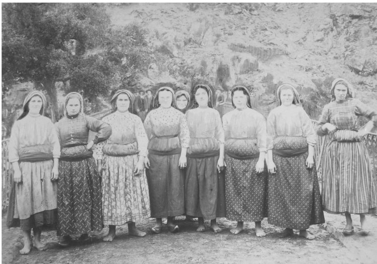
Figure 1. Concrete workers on the Luiz Bandeira Bridge over the Vouga, 1909 (IFA/CAA).
