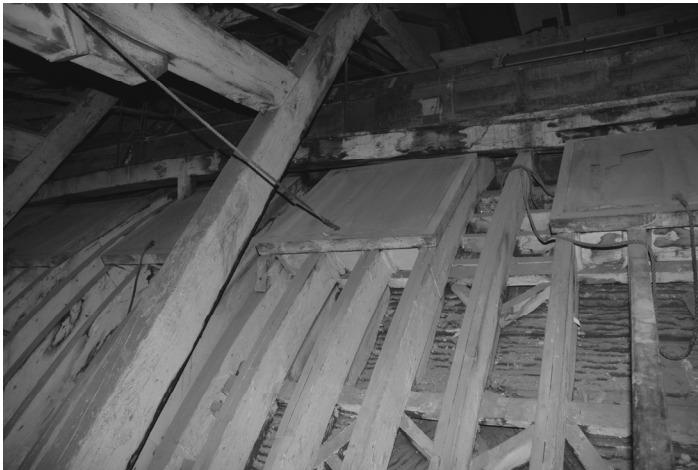
Figure 13. Flaps above air outlets
