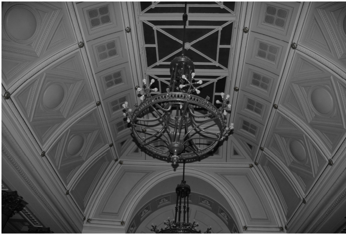
Figure 12. Court ceiling showing air outlets
