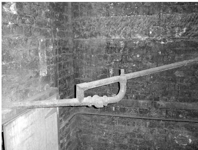
Figure 11. Location of gas jet at base of extract shaft
