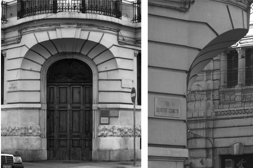
Figure 10. The trompe of the INCIS building
