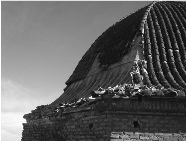
Figure 8. San Jaime Archpriestial of Vila-Real. Exterior view before restoration.
