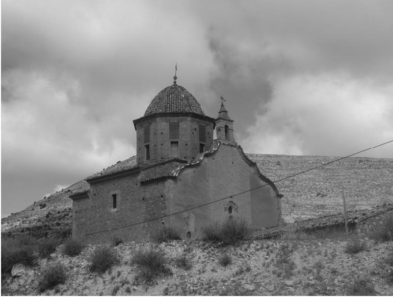
Figure 5. San Marcos Chapel. Olocau del Rey. General Exterior View.
