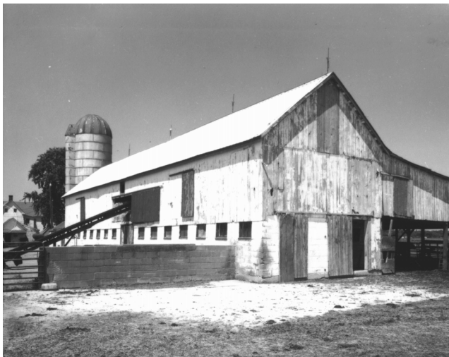
Figures 12 and 13. Examples of two different roof types for dairy barns. CHAD Collection.
