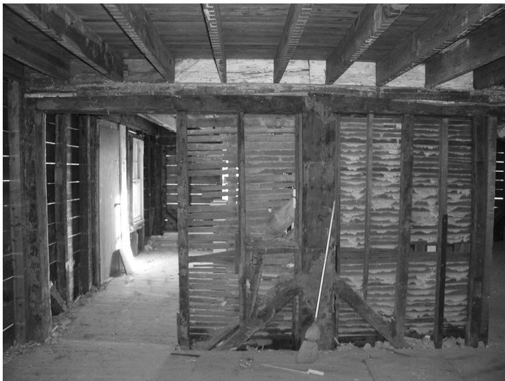
Figure 2. Framing visible in Willis-Ashton house. CHAD Collection.
