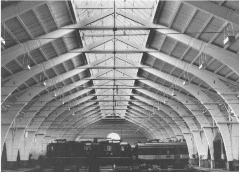
Figure 11. Railway Engine Shed in Bern 1911, photograph recent ( Müller 2000,p 72)
