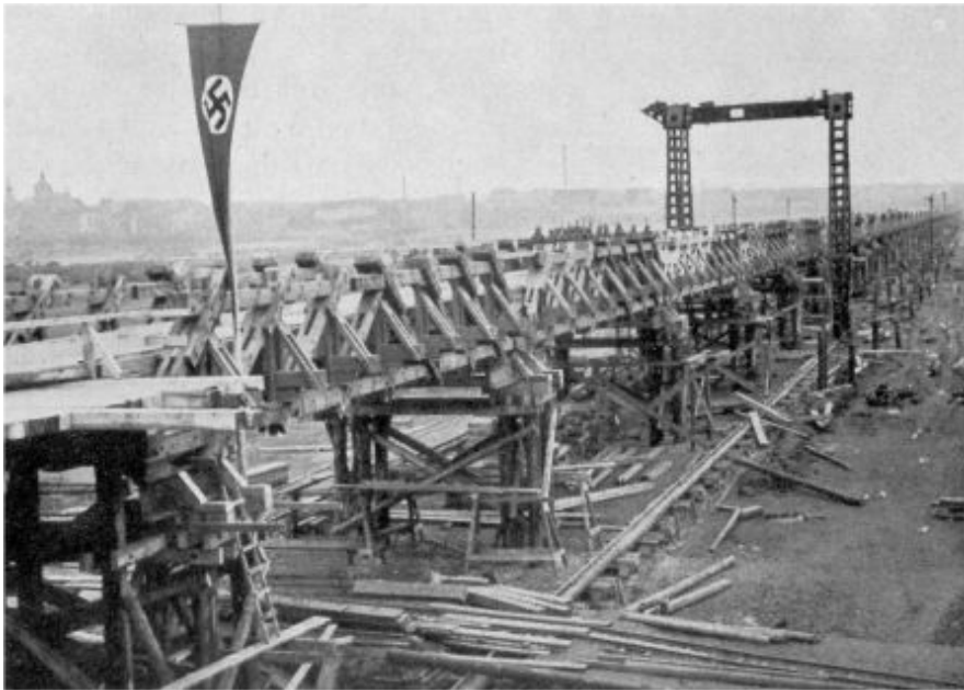
Figure 7. Auxiliary war bridge in Russia 1941 (Stoy 1942, p 135)
