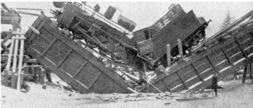
Figure 6. Fatal test loading of a reused plain beam 1919( Barz 1943, p 108)
