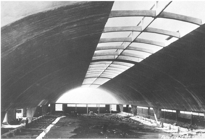
Figure 8. Shower and dressing hall in Serbariu mine site: a whole reinforced concrete barrel vault (AEM)
