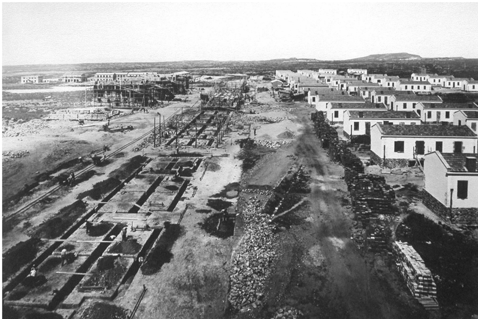
Figure 3. Aerial view of the building site with tipping wagons, groundworks and just finished houses, 1939 (AEM)
