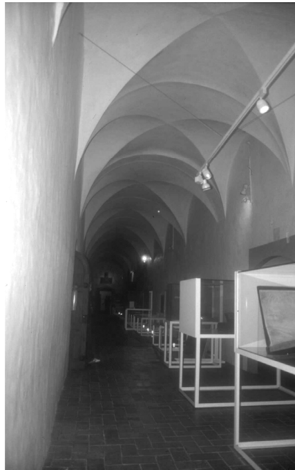
Figure 15. Interior of the sick ward, covered with a Renaissance vault in 1569.
