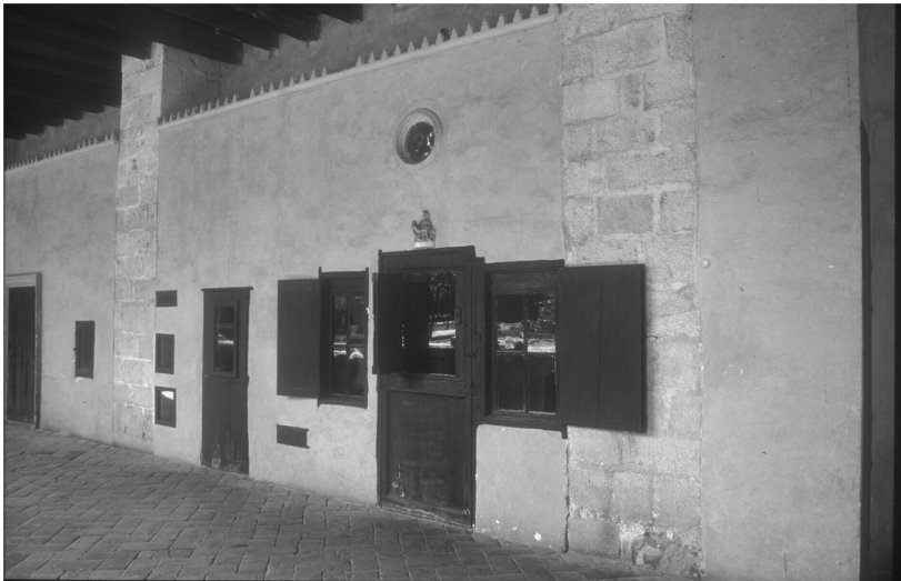
Figure 12. Private cells built between the buttresses of the dormitory. Cell of the Pieti.
