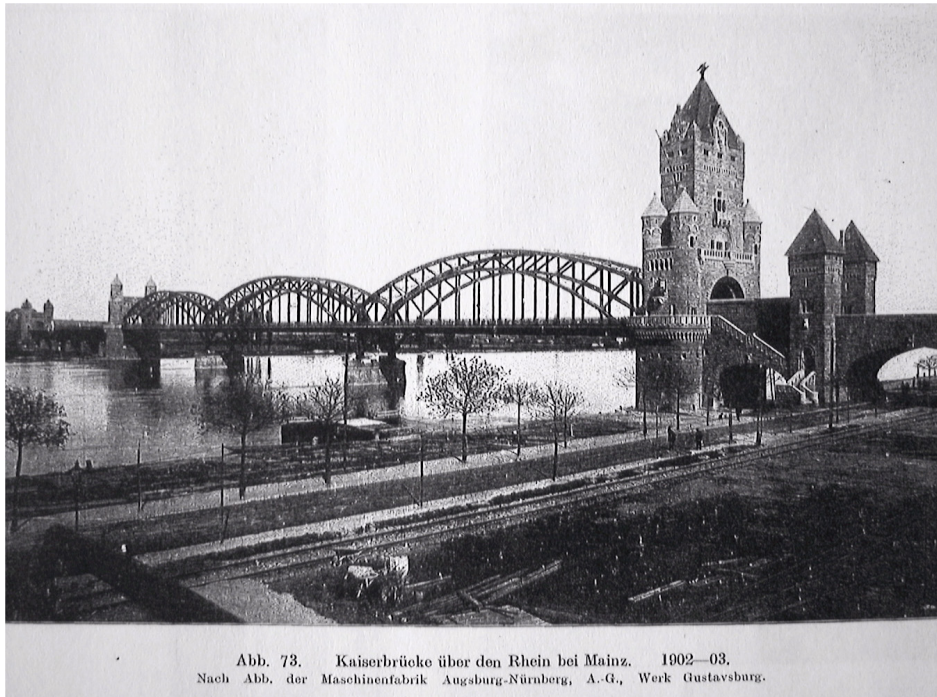
Figure 1. Kaiser Bridge near Mainz
