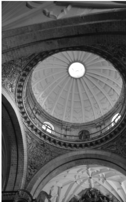
Figure 14. Juan Bautista Egidiano, Cuzco, church of La Compañía, interior detail of dome and rib vaulting over apse, 1651-68 (photo: H. Rodríguez-Camilloni).
