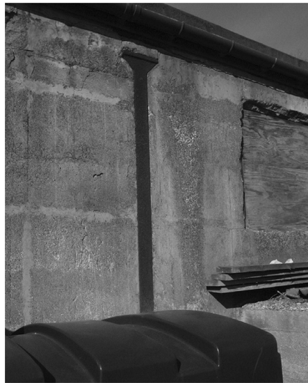
Figure 9. Detail of cast iron column in concrete panel wall (March 2004).
