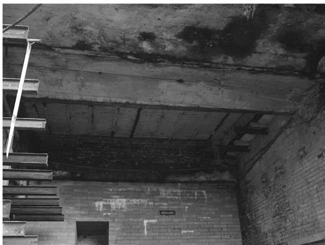
Figure 7. Concrete floor supporting Myrtle Road houses (March 2004).
