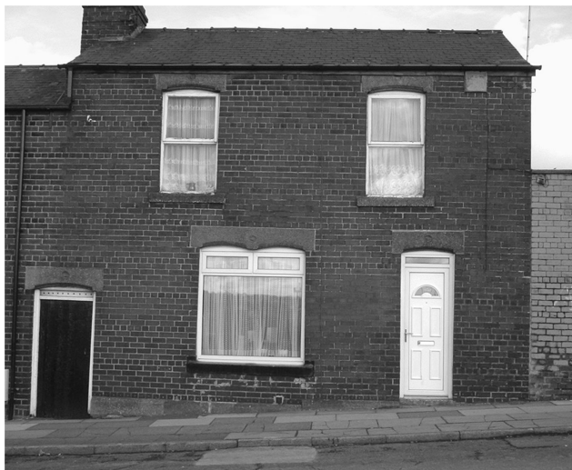
Figure 3. Myrtle Road House (March 2004).
