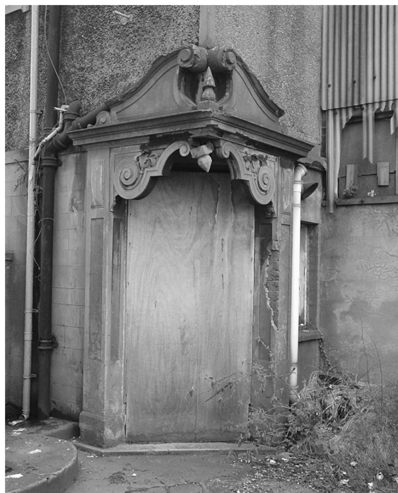
Figure 4. Decorative Plaster on doorway behind Queens Road frontage (March 2004)
