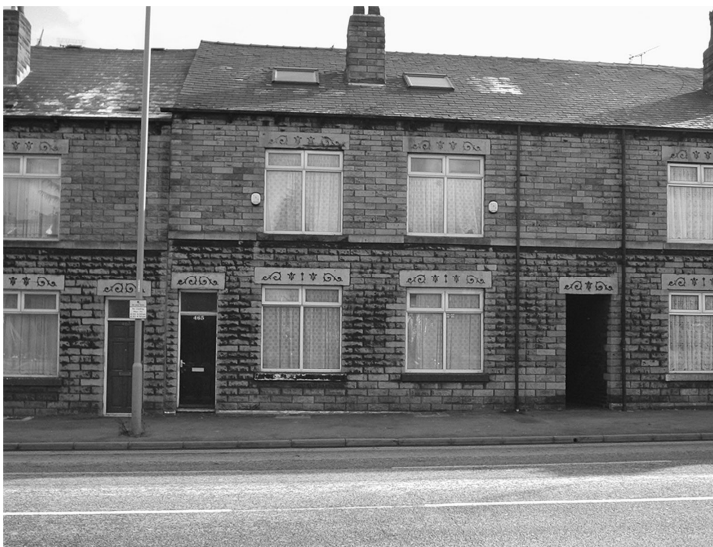
Figure 1. Houses at North West end of Queens Road terrace (March 2004).
