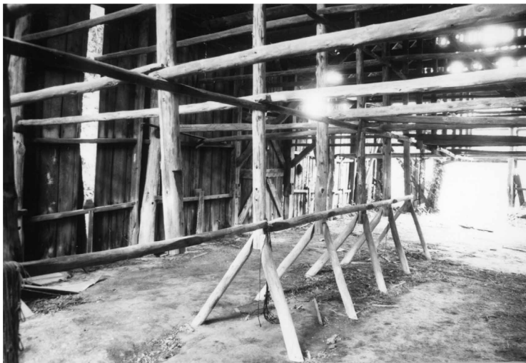
Figure 4. The interior scaffolding and “rooms” at the earthfast-constructed Bond Farm Tobacco Barn.
