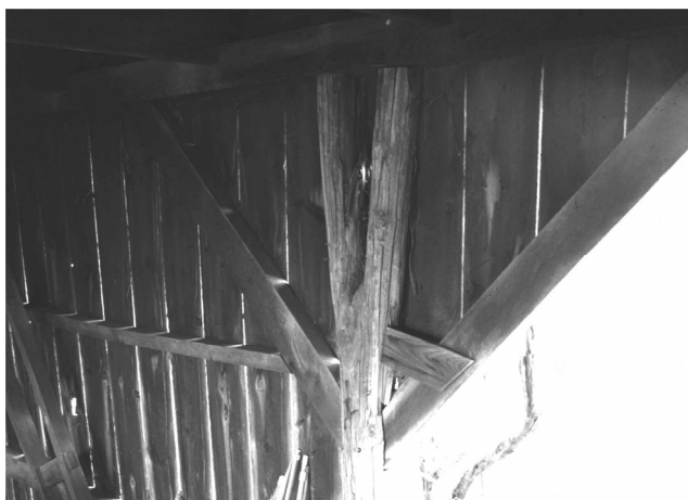
Figure 8. Forked post or “cratchet” at Jutland Farm.
