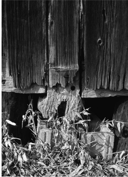
Figure 3. Earthfast post that has since been propped up by cinder blocks. Note the interrupted sill.
