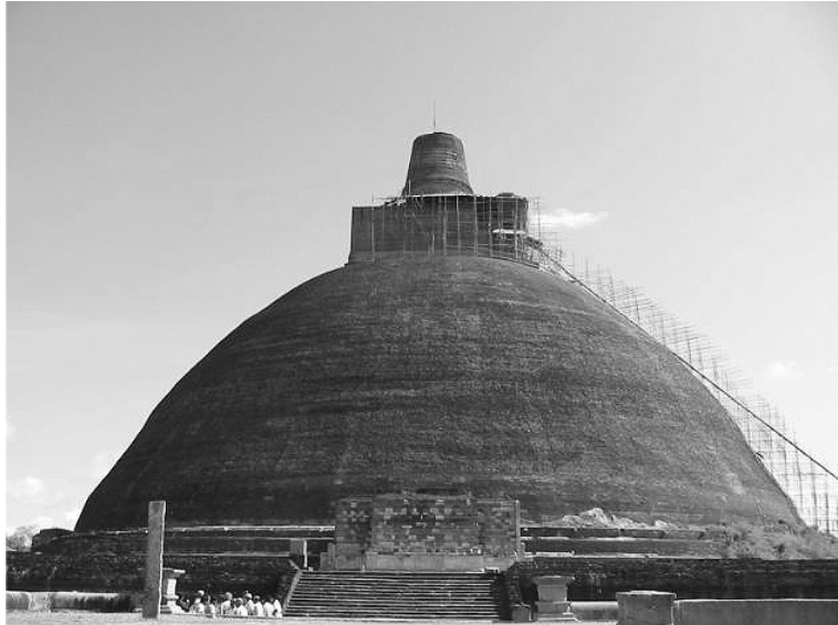
Figure 2. Jetavana stupa under conservation (height = 70.7 m, base diameter = 111.9 m)
