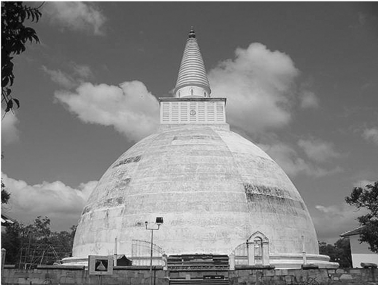
Figure 10. Mireseveti stupa after full restoration (height = 43 m, base diameter = 54 m)
