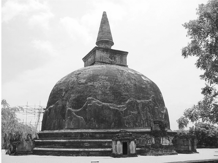
Figure 7. Kirivehera (height = 24.4 m, base diameter = 25.6 m) showing thick original plaster
