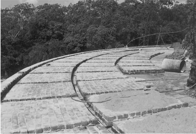
Figure 9. Mireseveti stupa restoration – new brickwork and groves for RC beams
