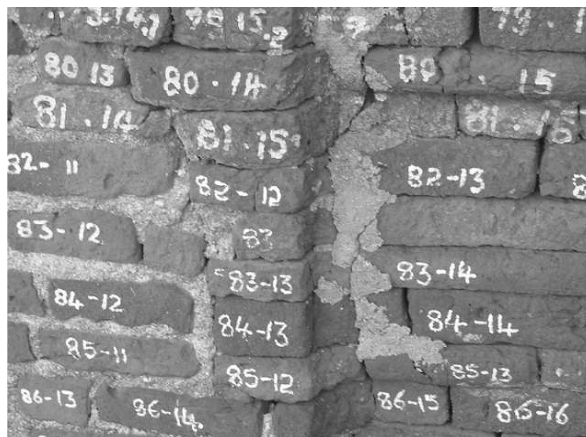
Figure 6. Comparison of ancient and British era brickwork in Jetavana
