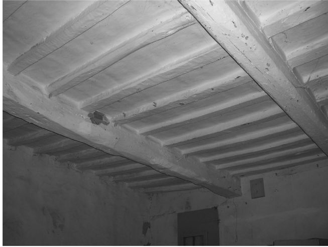
Figure 6. Interior showing the timber floor system.
