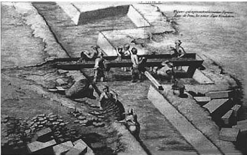
Figure5. Method where caissons are filled in situ (Forest de Belidor, B. 1729)
