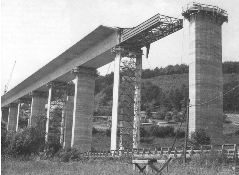
Figure 14. The incremental launched Taubertstalbrücke still needed intermediate supports (Wittfoht 1972, Bild 341)
