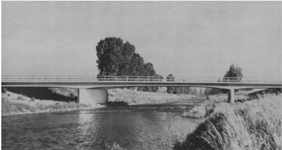
Figure 5. Elzbrücke in Emmendingen (Mörsch 1958, Abb. 97)
