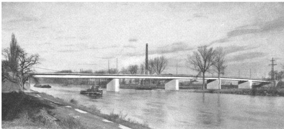
Figure 7. Neckarbrücke at Neckargartach (Mörsch 1958, Abb. 261)
