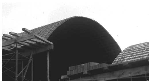
(a) Removal of formwork
