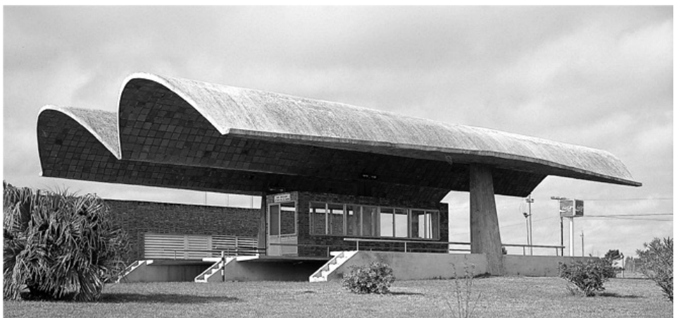
Figure 2. Double cantilever free-standing vault, Refresco del Norte, Uruguay (V del Amo)
