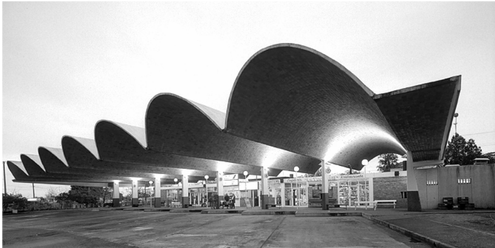
Figure 1. Free –standing barrel vault Bus Station Salto, Uruguay (V. del Amo)
