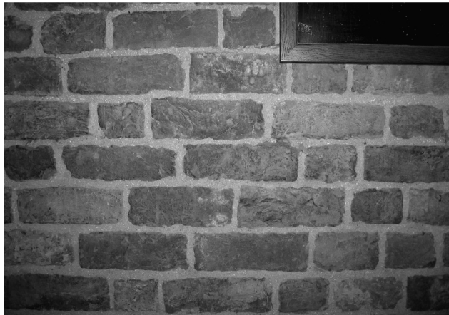
Figure 2. Gravensteen, Leiden; monk bond in the west wall, about 1200 (photograph by E. Orsel).
