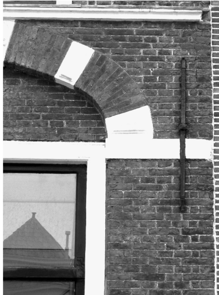
Figure 9. No. 129, Rapenburg, Leiden, 1630; brickwork with closer corner bond and three-quarter bat bond at windows (photograph by E. Orsel).
