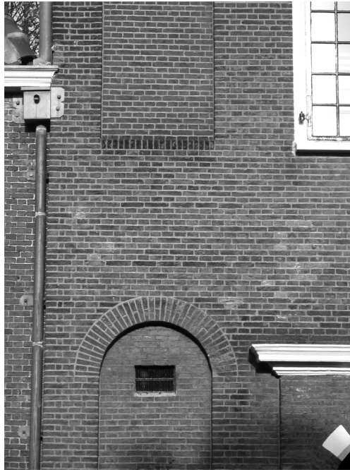
Figure 11. No. 21, Kloksteeg, Leiden, Pesijnhof, 1683; brickwork with closer and three-quarter bat corner bonds (photograph by E. Orsel).
