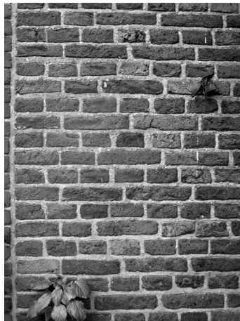
Figure 8. No. 7, Vijfde Binnenvestgracht, Leiden, 1588; three-quarter bat corner bond (photograph by E. Orsel).
