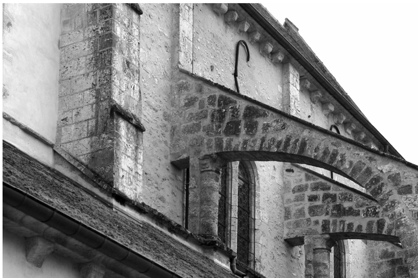
Figure 4. Detail of flying buttress at Donnemarie (photo: Tallon)
