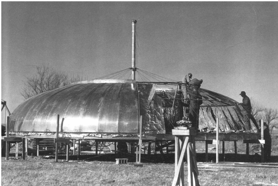
Figure 10. Assembling the Dymaxion House, Wichita 1946 (Krause 1999)
