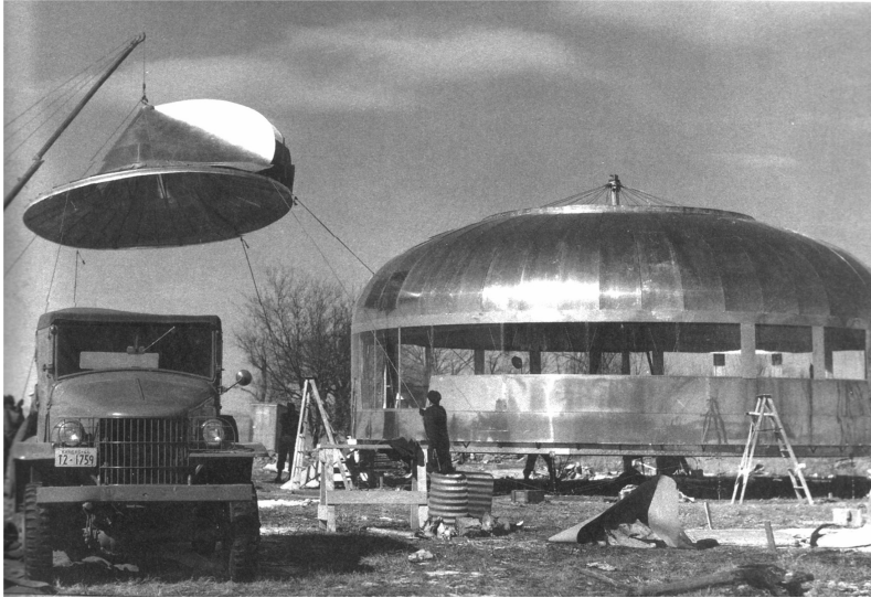
Figure 11. Assembling the Dymaxion House, Wichita 1946 (Krause 1999)
