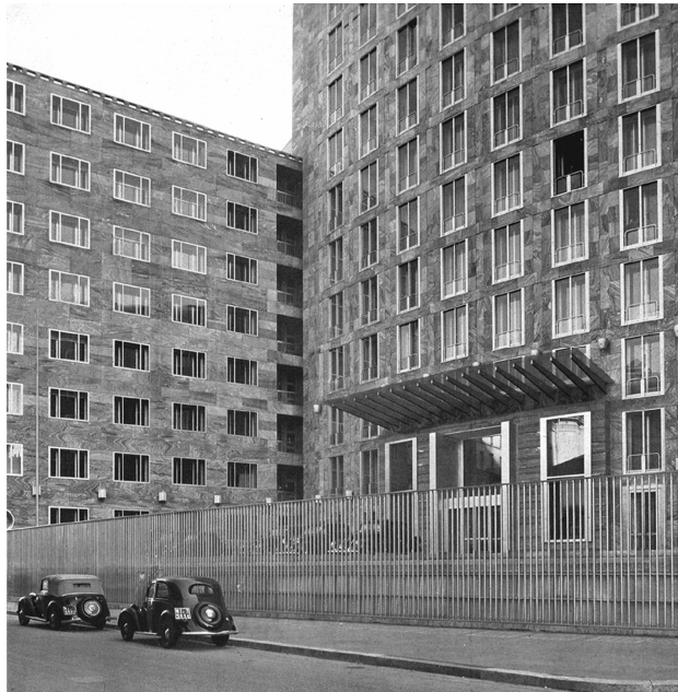
Figure 11. View of the Main Entrance from via Moscova (Casabella 1939)
