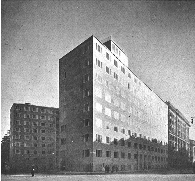
Figure 1. View of the Building (Casabella, 1939).
