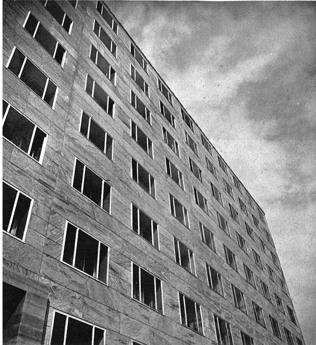
Figure 8. The Exterior Aluminium Windows of the Side Volumes (Il palazzo 1938).
