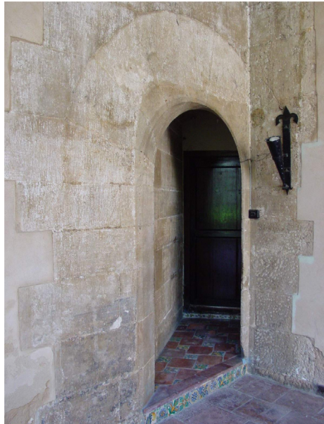
Figure 10. Skew door of the kitchen at the cloister in Trinity convent, Valencia.
