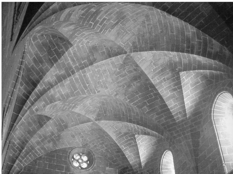
Figure 1. Vault in the Royal Chapel in the Santo Domingo convent (Valencia), Francesc Baldomar, 1439- 1451.
