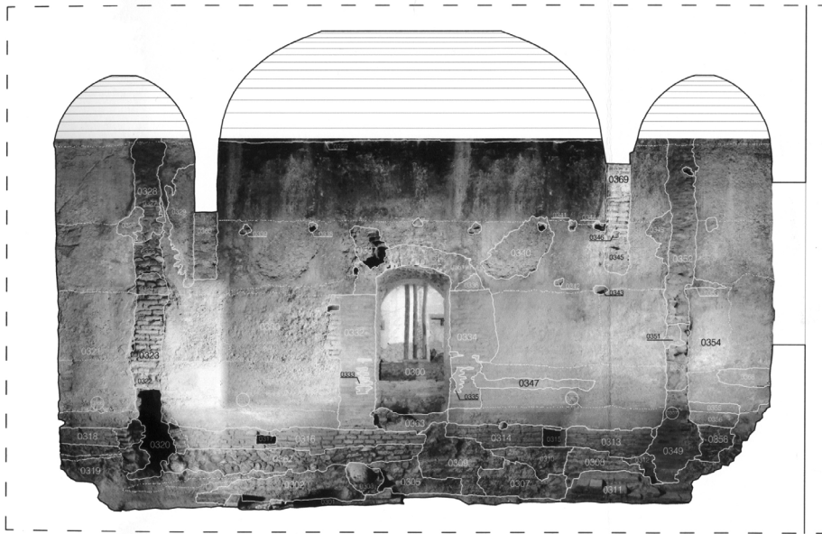
Figure 5. Stratigraphic study of the South wall of the caldarium
