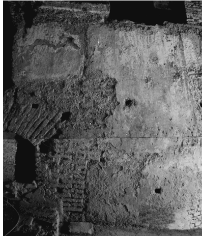
Figure 7. Pisé-de-terre with an arch made of bricks, both built simultaneously
