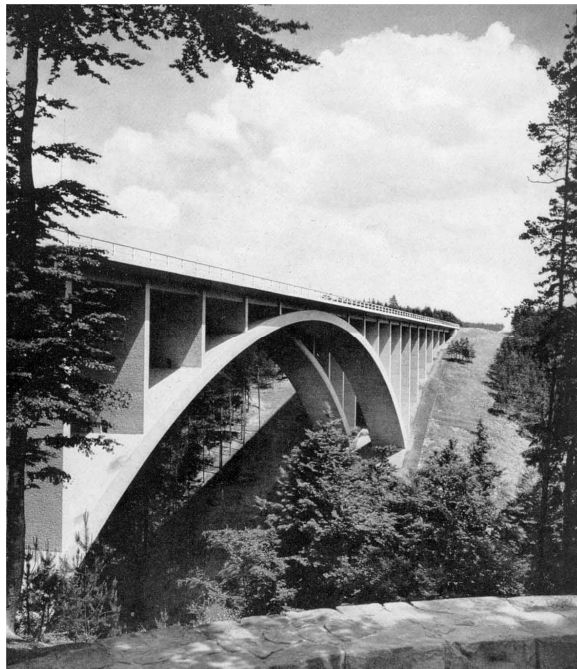
Figure 14. Paul Bonatz (architect), Teufelstalbrücke near Hermsdorf, 1936-38 (Bonatz and Leonhardt 1951, p. 82)
