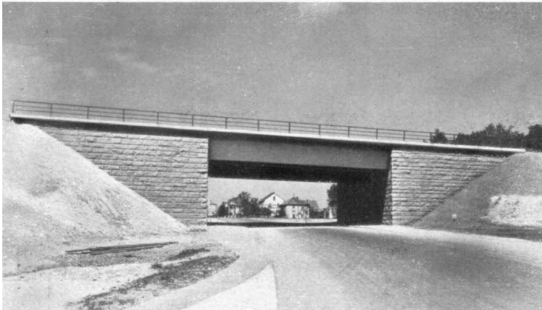
Figure 11. Solutions for an overpass and an underpass from the OBK Dresden, ca. 1938 (Buschmann 1939, p. 25)
