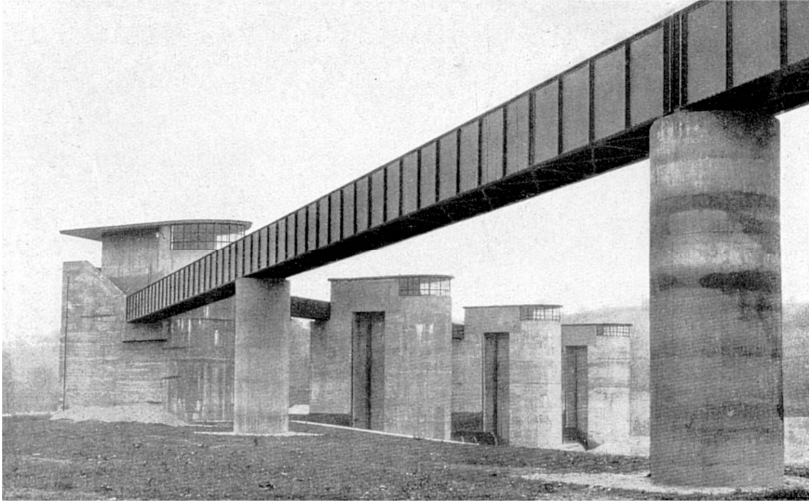
Figure 1. Paul Bonatz (architect), Neckar barrage at Horkheim, 1927-29 (Graubner 1931, p. 24)
