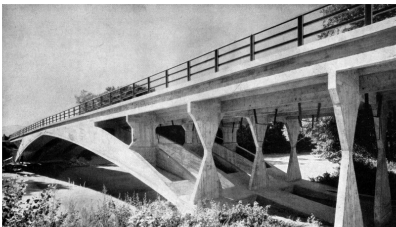
Figure 13. Robert Maillart, Bridge over the Arve River at Vessy, 1934-36 (Bill 1949, p. 119)
