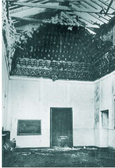
Figure 3. State of the Hunters Lounge and its panelwork after the fire in 1936. In the photo we see how a great part of the panelwork remained, although today we do not know what has happened to it.
