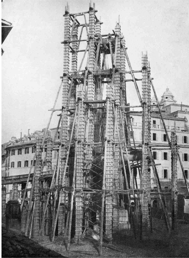
Figure 8. Scaffold used to raise of the Immaculate Conception column in Piazza Mignanelli (1856)
