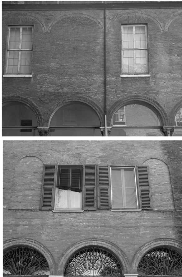
Figure 5. Traces of modifications to the side balconies of the courtyard and traces of the upper arcade facing the garden
