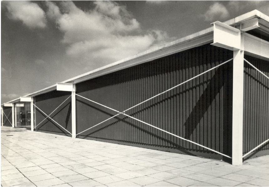
Figure 2. The Reliance Controls factory, Swindon, England, 1967. Team 4, architects; Anthony Hunt Associates, engineers. This was the first building of British High Tech.
