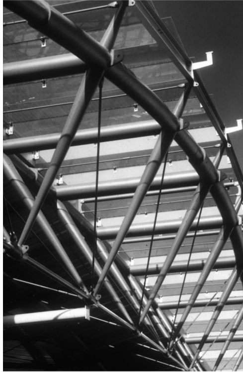
Figure 10. The space trusses that formed the principal structural elements of the Waterloo Terminal have a highly complex 3-dimensional form.
