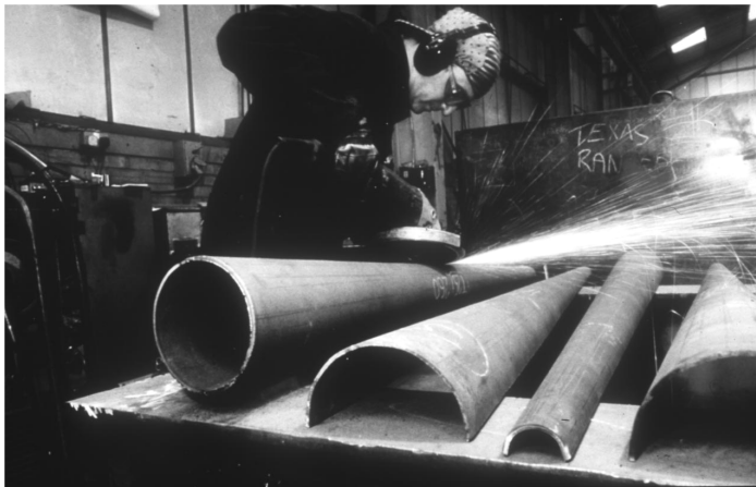
Figure 13. The tapered hot rolled scantlings of the principal trusses were fabricated in two halves, by a brake-press technique, which were then welded together.
