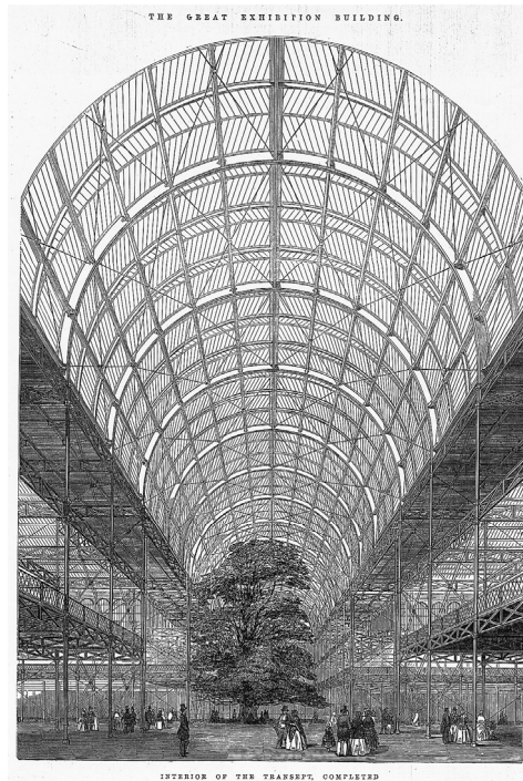
Figure 6. Crystal Palace, interior of the newly completed transept ( The Illustrated London News , 25 January 1851)
