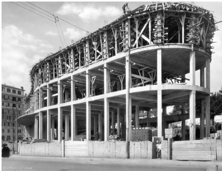
Figure 9. Post Office Building in piazza Bologna, Rome, in construction. Mario Ridolfi, 1933-1935 (Poretti 1990)
