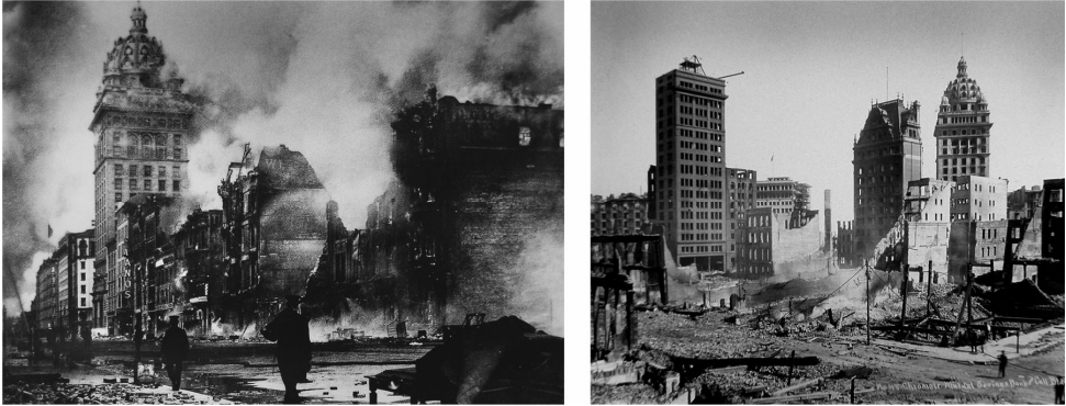
Figure 7. San Francisco in 1906 showing Chicago Frame buildings that burned out but remained standing. All of the taller buildings in these images are still extant in 2006. (Bancroft Library)
