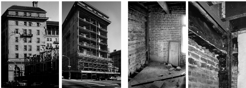
Figure 9. (L) The Oakland Hotel showing damage to façade, and later during repairs. (R) The Touraine Hotel, Oakland, California showing masonry exterior infill during upgrade work.
