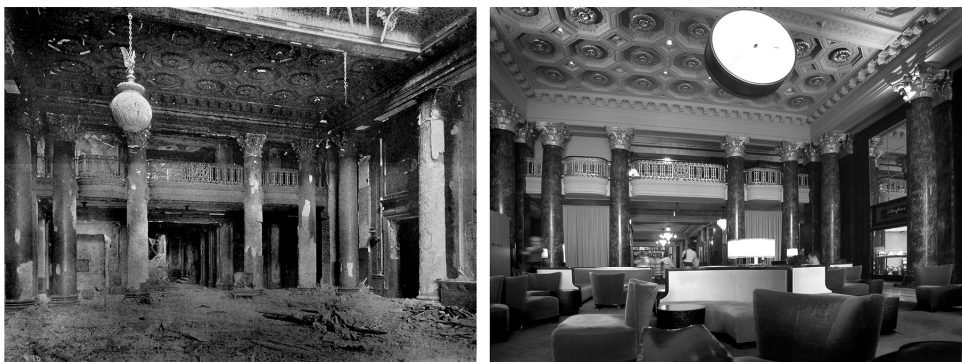
Figure 8. St Francis Hotel lobby after the 1906 earthquake and fire, and same space still extant 100 years later. (Roebling, 1906)
