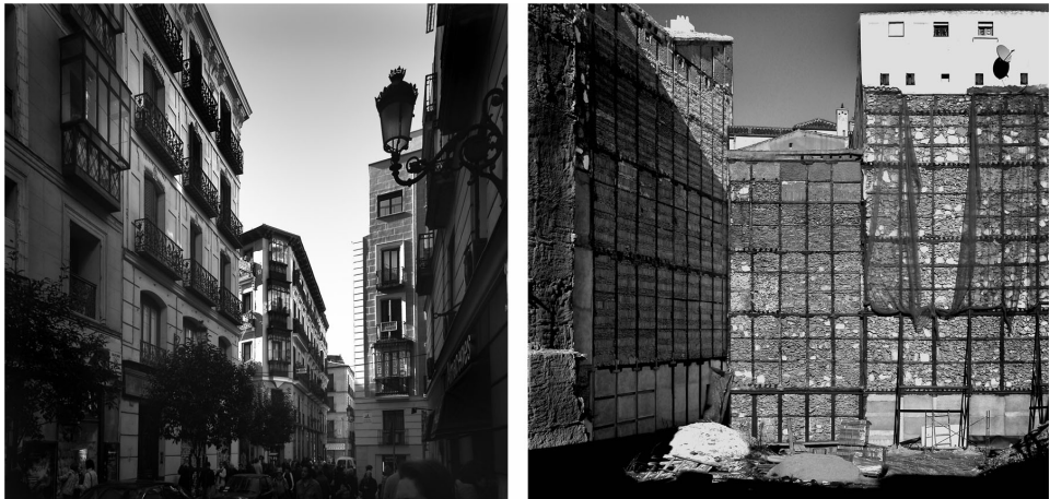
Figure 12. Historical center, Madrid showing front façades and infill masonry timber frame construction revealed on rear walls after demolition of adjacent structures in 2002.
