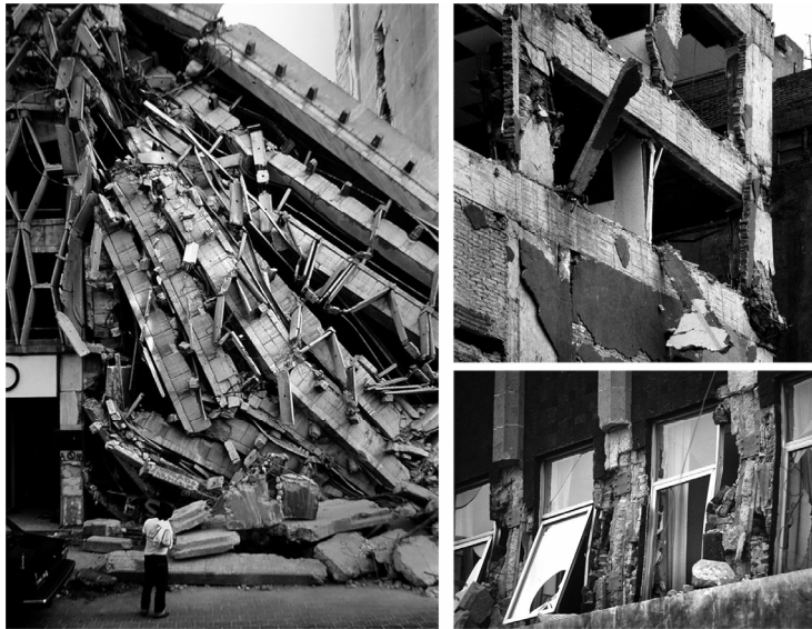
Figure 11. Mexico City 1985 earthquake: (L) Collapsed RC Parking garage. (C) RC frame showing column damage and loss of infill. (R) Bent steel frame in ca.1940 building with too little masonry to help.
