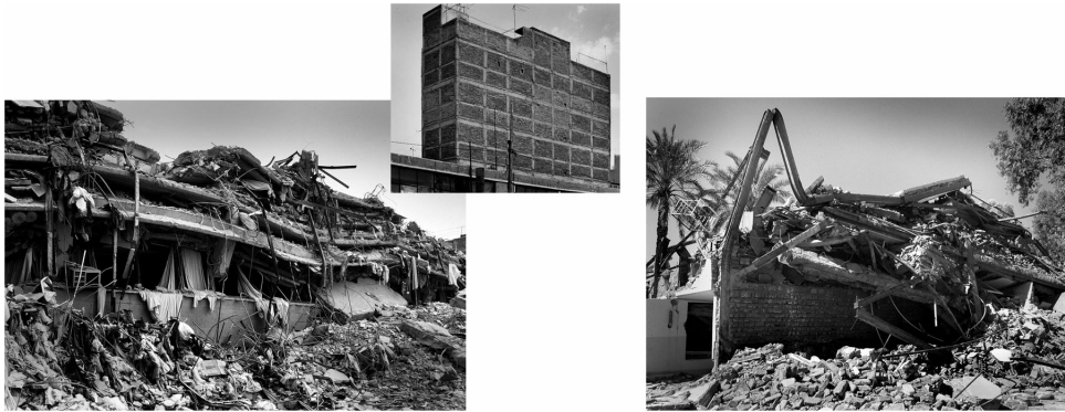
Figure 2. (L) Juarez Hospital after 1985 Mexico City earthquake with neighboring (C) undamaged infill-frame RC building. (R) Steel building after 2003 Bam, Iran earthquake.
