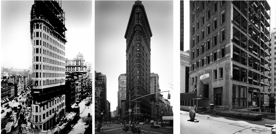
Figure 4. (L) Flatiron Bldg (1902), NYC. Masonry façade with construction beginning on upper floors at same time as at foundation (vazyvite.com). (C) Flatiron Bldg. (R) 343 Sansome, San Francisco.
