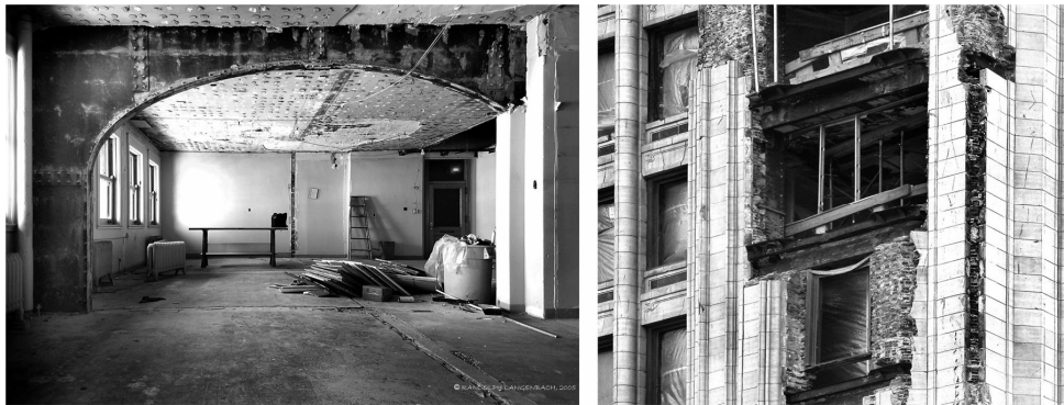
Figure 6. (L) Portal arch wind bracing in Monadnock Building, South Half (1891-3). (R) Cladding on 90 West Street (1907) damaged by World Trade Towers collapse showing steel shelf angles.
