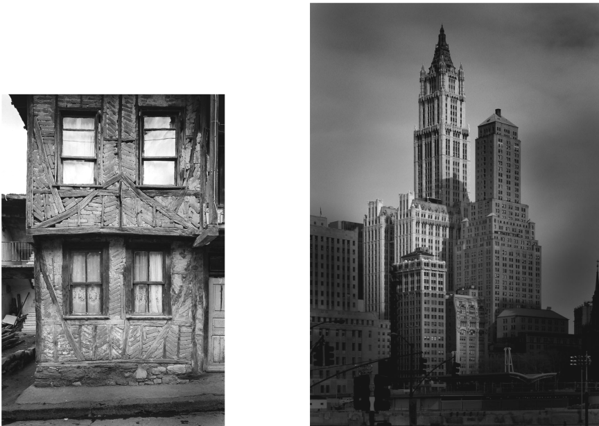
Figure 1. (L) Undamaged hımış construction in Gölcük, Turkey. (R) 1913 Woolworth Tower by Cass Gilbert, is now the tallest building in Lower Manhattan after the collapse of the World Trade Towers.
