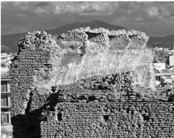
Figure 11. Argos, Greece. Detail of remains of vault of main hall showing voids divided by low walls over haunch.
