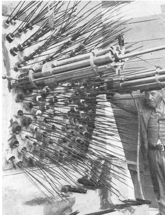
Figure 14. Barredo System .Torroja,E. 1955.
