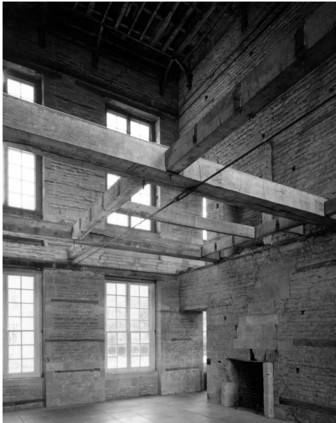
Figure 1. Interior of unfinished wing at Boughton House, showing bond timbers
