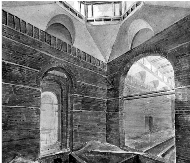
Figure 11. Drawing by one of Sir John Soane's pupils of construction in progress at Dulwich showing bond timbers (Vol.18/22)
