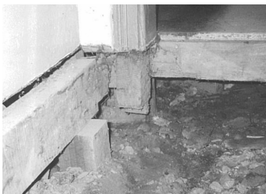
Figure 10. Tenoned end to centre wall stud
