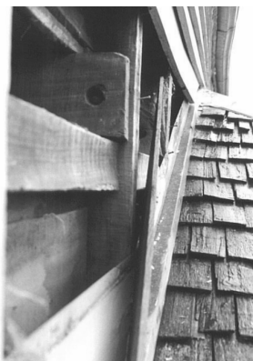
Figure 9. Rebated wells in floor joist ends.
