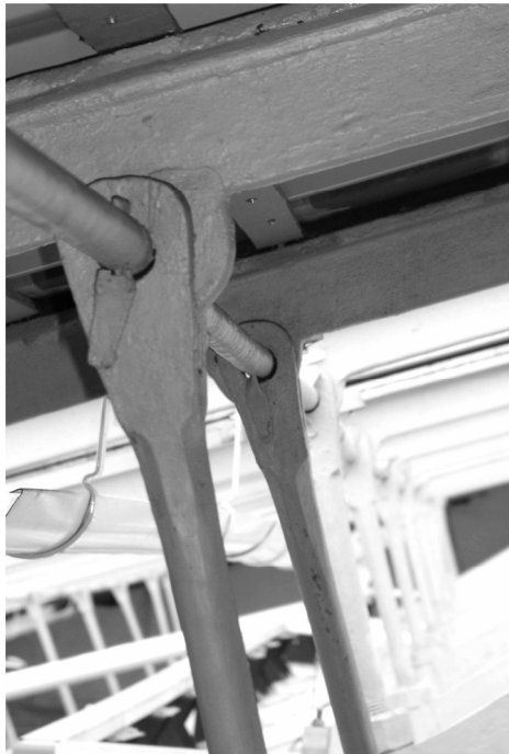
Figure 13. Forged eye of a rafter with an offset (Nobel 1844)
