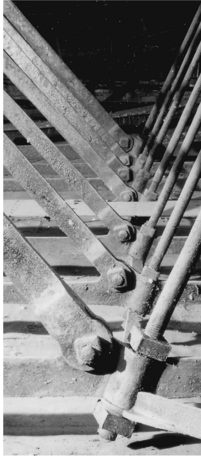
Figure 5. Connections: strut with tread and nuts and the branched bottom cord with bolts
