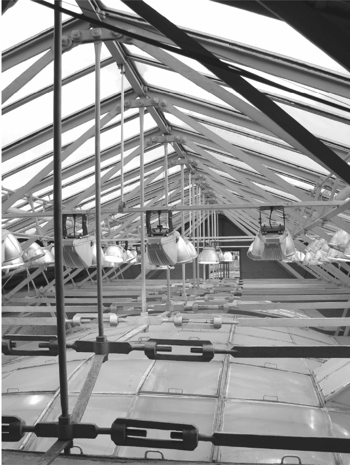
Figure 3. Roof trusses over the exhibition halls with roof light
