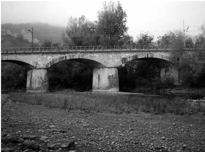
Figure 10. Oblique bridge near Vergato on the Porrettana railway
