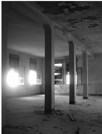
Figure 11. Colonia Marina Fascista in Rimini: concrete columns in the big rooms facing the sea
