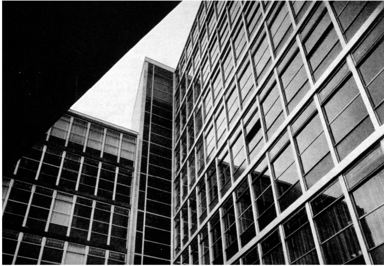
Figure 2. Photograph of the curtain wall (photograph by De Jongh, Bulletin Technique de la Suisse Romande , n° 25 1953)
