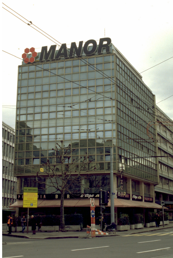
Figure 8. Photograph of the building (F. Graf, March 2001)
