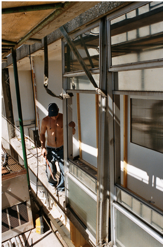
Figure 13. Panel being taken down (photograph by M. Thomann 2 September 2004)
