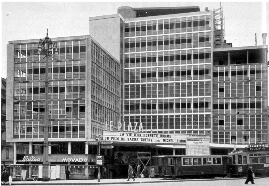
Figure 1. Photograph of the finished building (AS n°3 1953)
