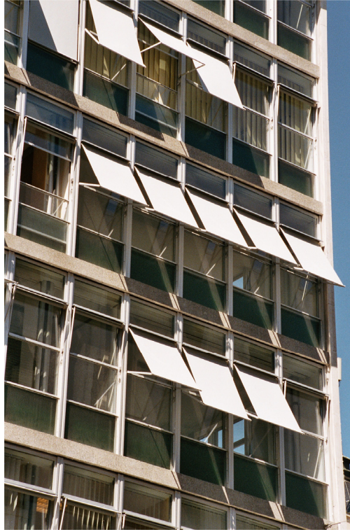
Figure 14. Replica panels being installed (photograph by M. Thomann 2 September 2004)
