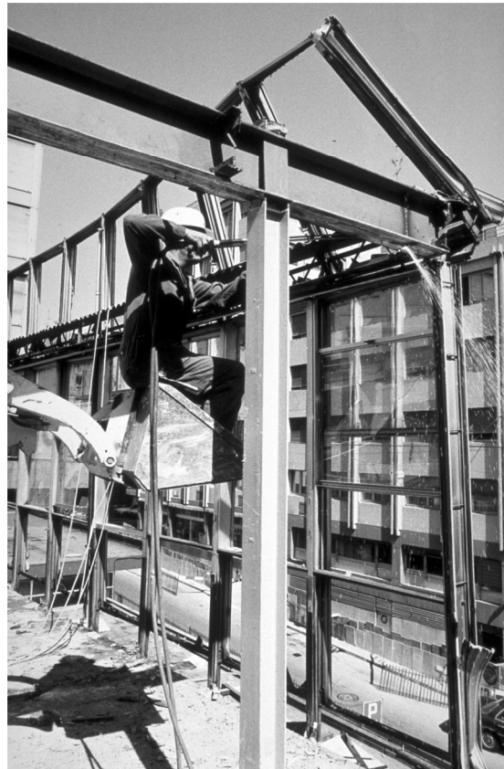
Figure 12. Photograph of the building during demolition (photograph by M. Oetli, September 1987)
