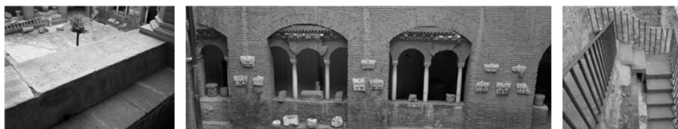
Figure 9. Details of new elements in travertine, breccia, peperino and metal
