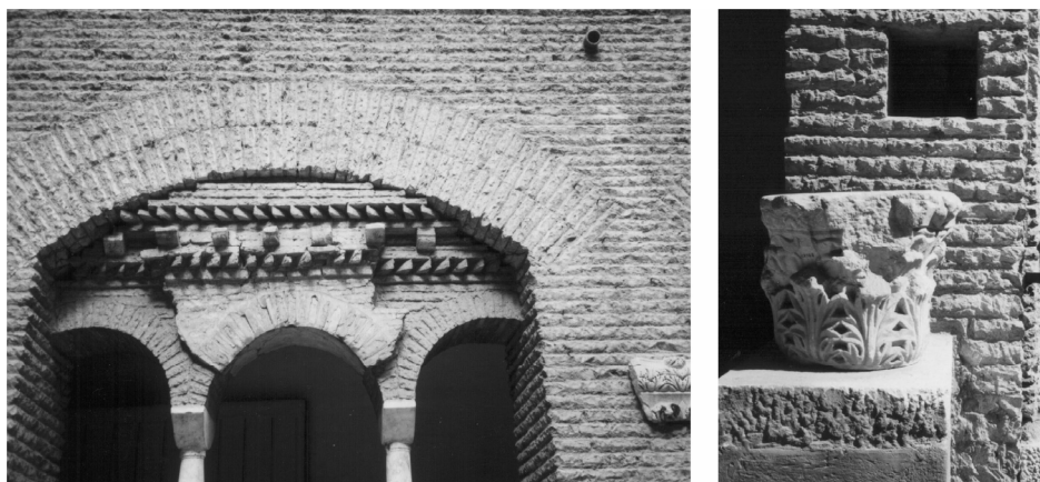
Figure 15. Details of the new breccia stone wall to the west side of the cloister, at ground floor level (author)
