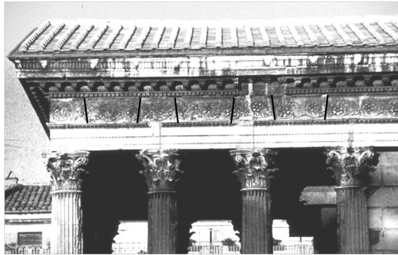
Figure 2. Entablature of the Maison Carrée in Nîmes. Highlighted in black are the joints between the pieces of the frieze, which form a flat arch unloading the monolithic architrave (photo. by the author)
