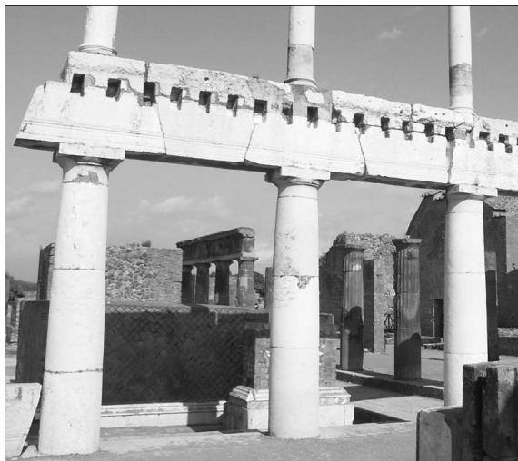
Figure 3. Entablature of the Forum of Pompeii, in which the architrave and frieze are joined to form the voussoirs of a flat arch (photograph by the author)
