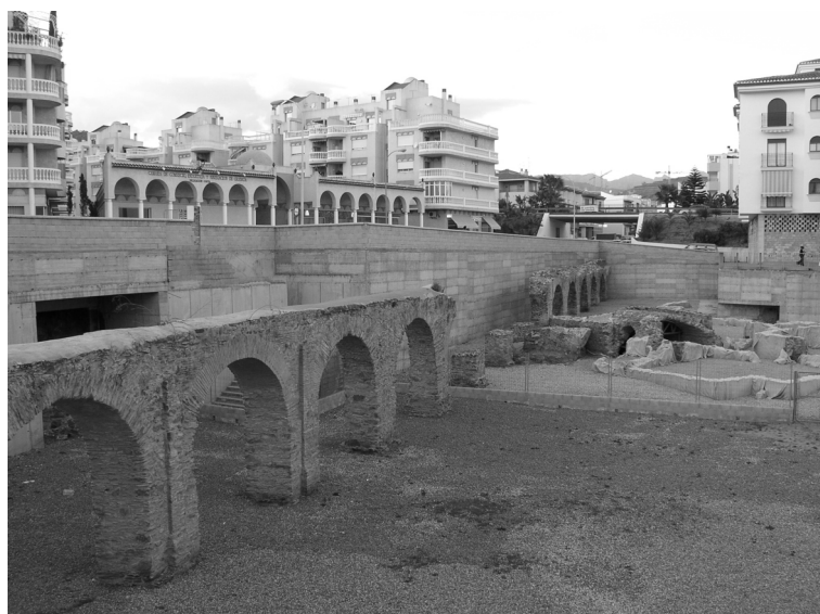
Figure 6. Venter of the siphon of the Almuñécar aqueduct.
