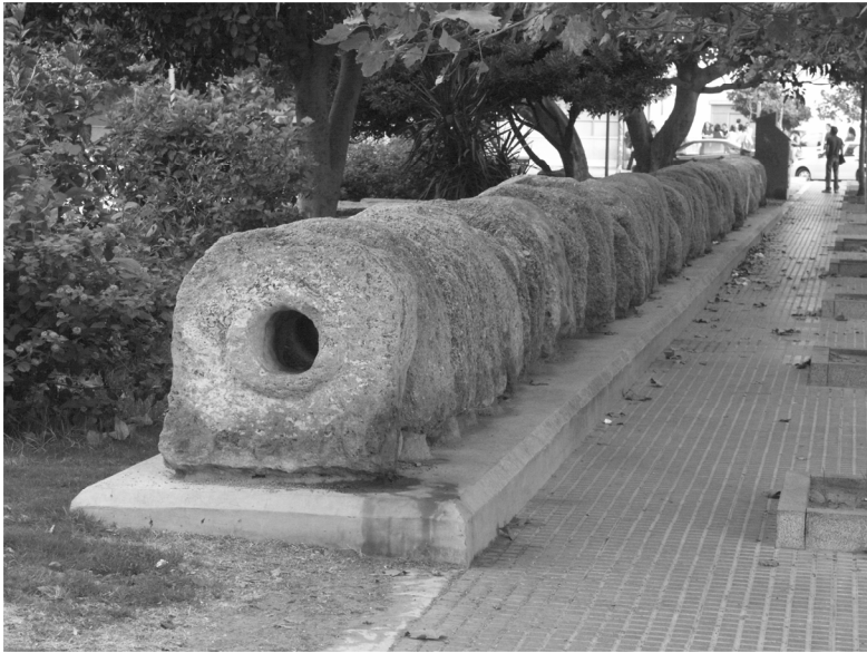
Figure 1. Pipeline of Gades aqueduct. Part of stone siphon.
