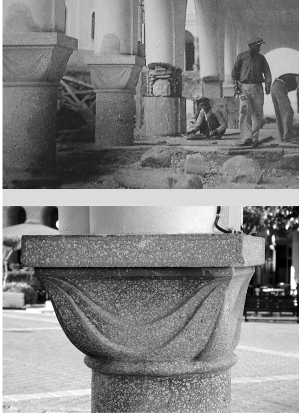
Figure 13. The New Market at Kos. A contemporary picture of the works), and detail of a concrete grit capital (Markoglu 1992).
