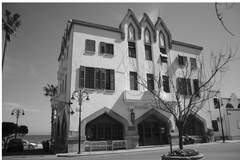
Figure 9. The Albergo Gelsomino in Kos. Tiles of "artificial" stone in the crowning gable.
